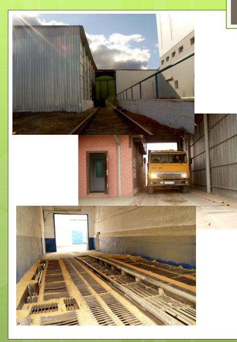
• The company has the ability to produce reception and ship products both by road and by rail. There are storage bins on the territory for receiving grain by road and rail with the subsequent movement of grain into loading elevators. There are warehouses with a total capacity of 10,000 tons of packaged product on the territory.
